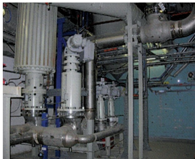
Site of the HK vault at Chooz A: before work – 2010
