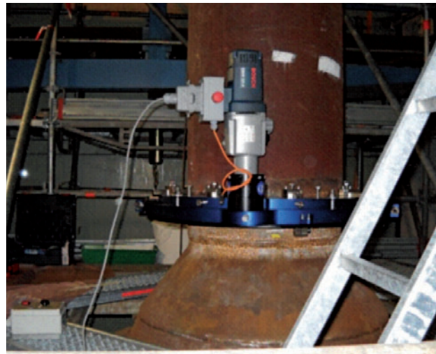
Preparation for the extraction of a steam generator at Chooz A – 2010
