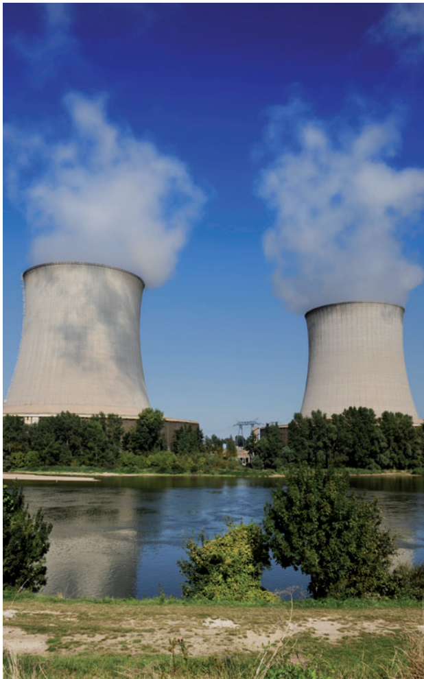
The Saint-Laurent-des-Eaux NPP viewed from the banks of the River Loire
