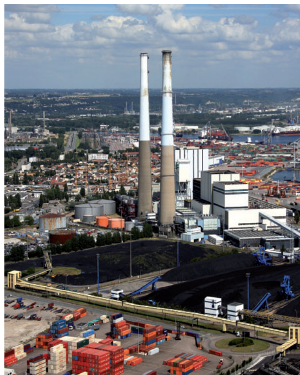
Aerial view of Le Havre thermal power plant
