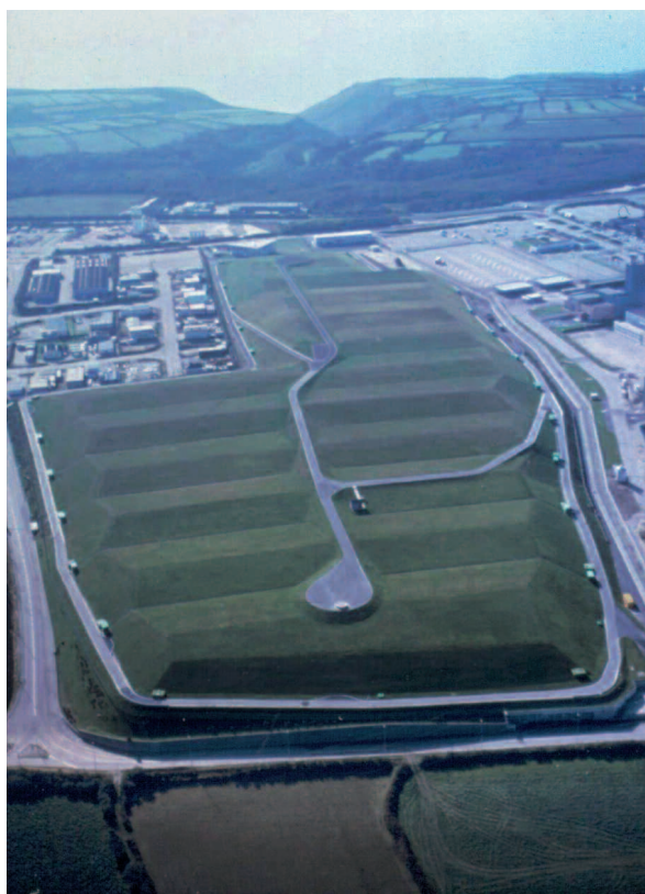
View of the Manche repository
