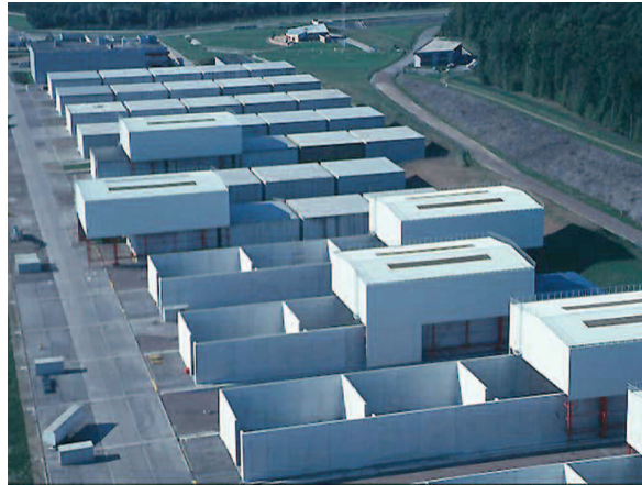
Disposal structures in the Aube repository
