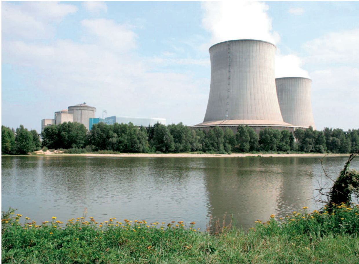
The Loire river at Saint-Laurent-des-Eaux (Loir-et-Cher département ): protecting the natural environment
