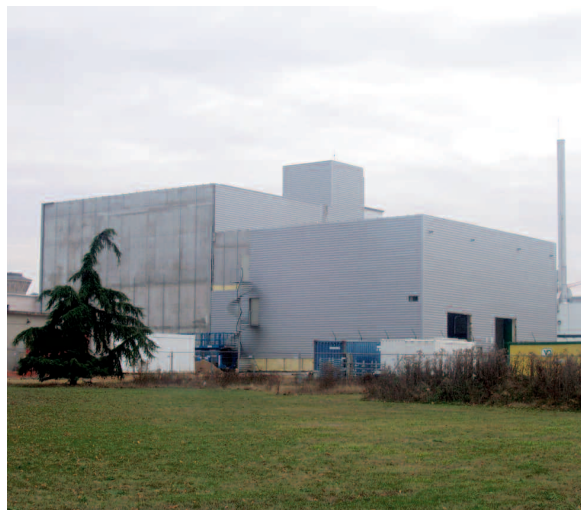
STELLA extension building in BNI 35 in Saclay (Essonne département)
