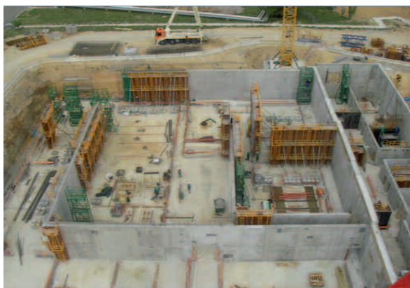
View of the MAGENTA facility construction site
