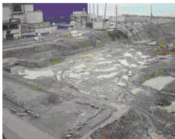
EPR construction site in Flamanville (Manche département) – August 2007: site preparation works
