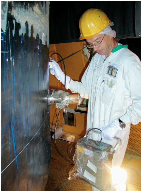
Ultrasonic inspection of a weld joint
