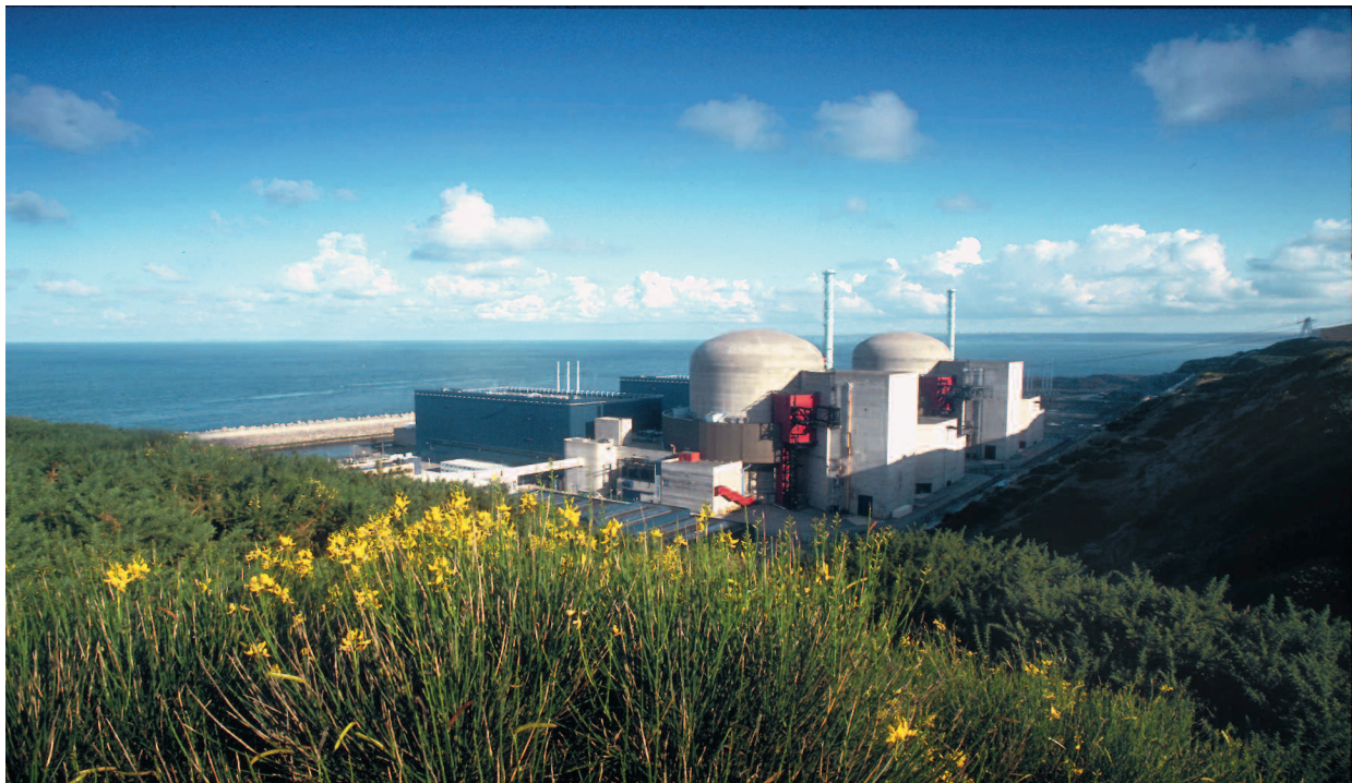
Flamanville nuclear power plant (Manche département)
