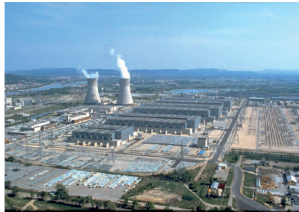
View of the EURODIF gaseous diffusion uranium isotopes separation facility on the Tricastin site
