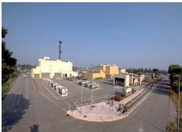
View of the TU5 installation on the Tricastin site
