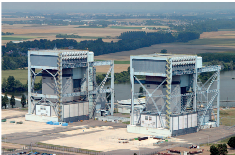
The two gas-graphite reactor units in the Saint-Laurent-des-Eaux nuclear power plant (Loir-et-Cher département)
