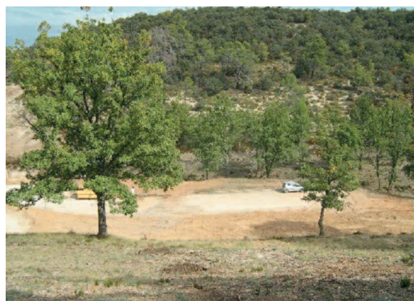
View of the HARMONIE reactor building (Bouches-du-Rhône département) in Cadarache after decommissioning
