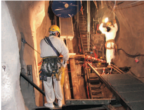
Operators working on decommissioning the CHOOZ reactor ventilation duct (Ardennes département)
