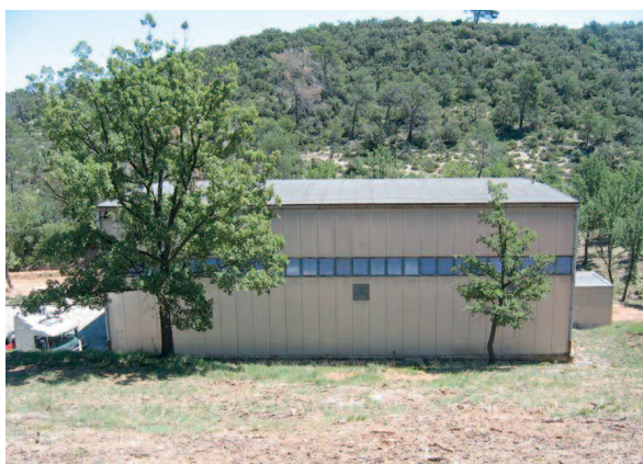
View of the HARMONIE reactor building (Bouches-du-Rhône département) in Cadarache before decommissioning
