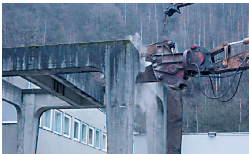
Chooz A — Demolition of the turbine hall
