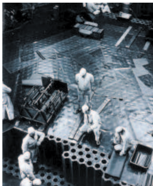
Graphite stack in a gas-graphite Uranium reactor
