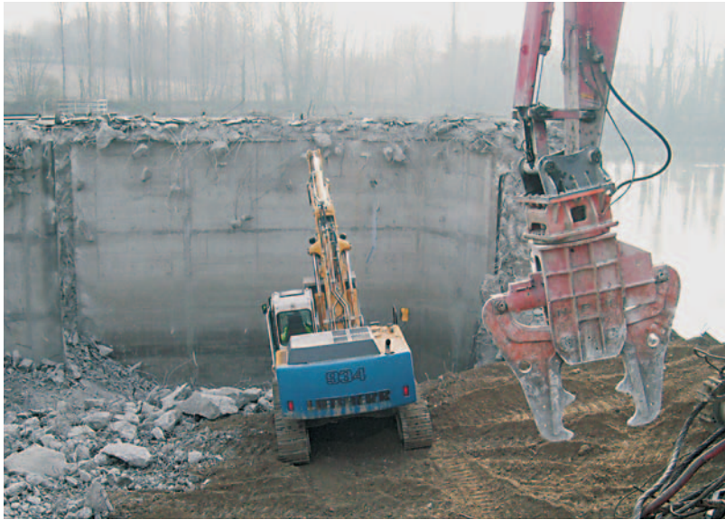
Bugey 1 — Demolition of the pump- ing station
