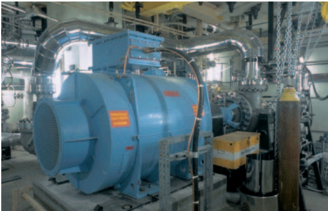
RRA pump on the N4 plant series
