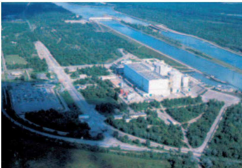
Fessenheim nuclear power plant
