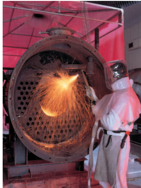
Dismantling of a nuclear installation
