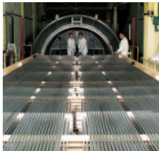
Tube installation in a steam generator
