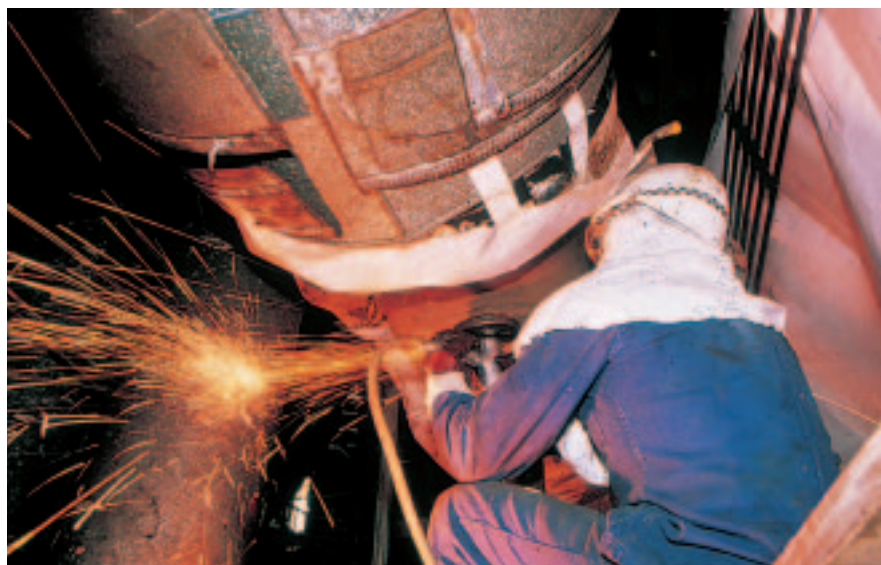
Welding job site
