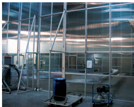
Installation of BNI 79 decay pits containment
