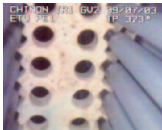
Tube installation in a steam generator
