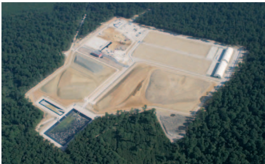
VLL waste repository
