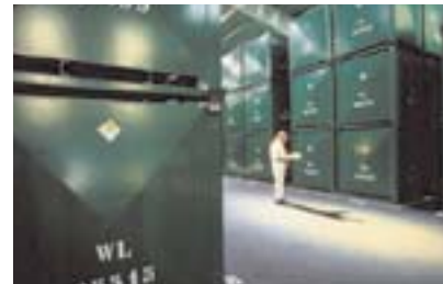
Uranium oxide interim storage
