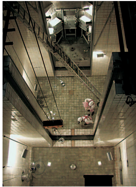
Mélusine — empty reactor pit
