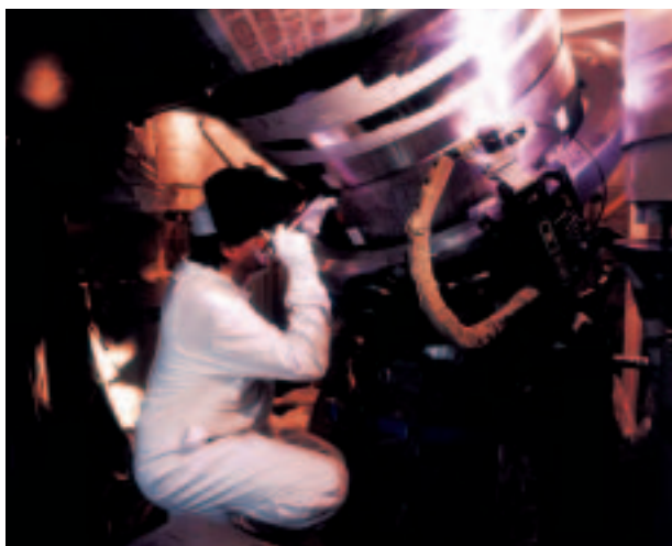
Welding operation during steam generator replacement
