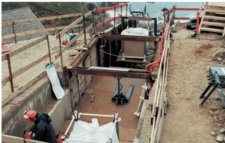
Demolition of concrete coating zone 2
