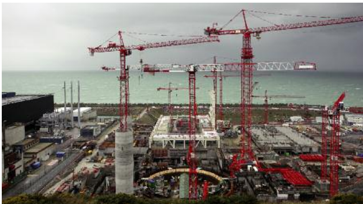
View of the future Flamanville 3 EPR reactor – January 2009
