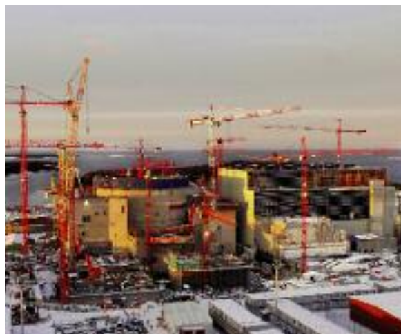
EPR worksite at Olkiluoto (Finland) – January 2009
