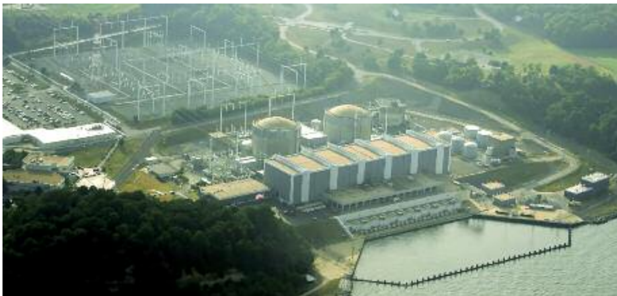
The Calvert Cliffs plant in Maryland, United States, was commissioned in 1975
