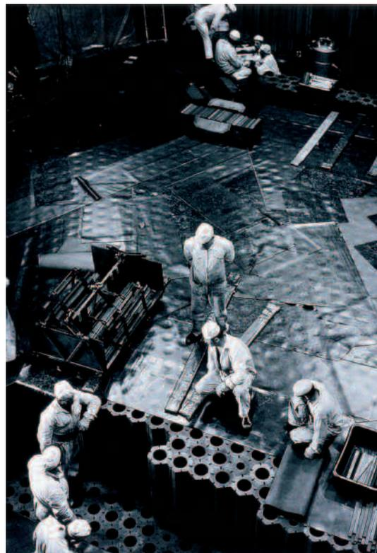
Graphite assembly in graphite gas reactor
