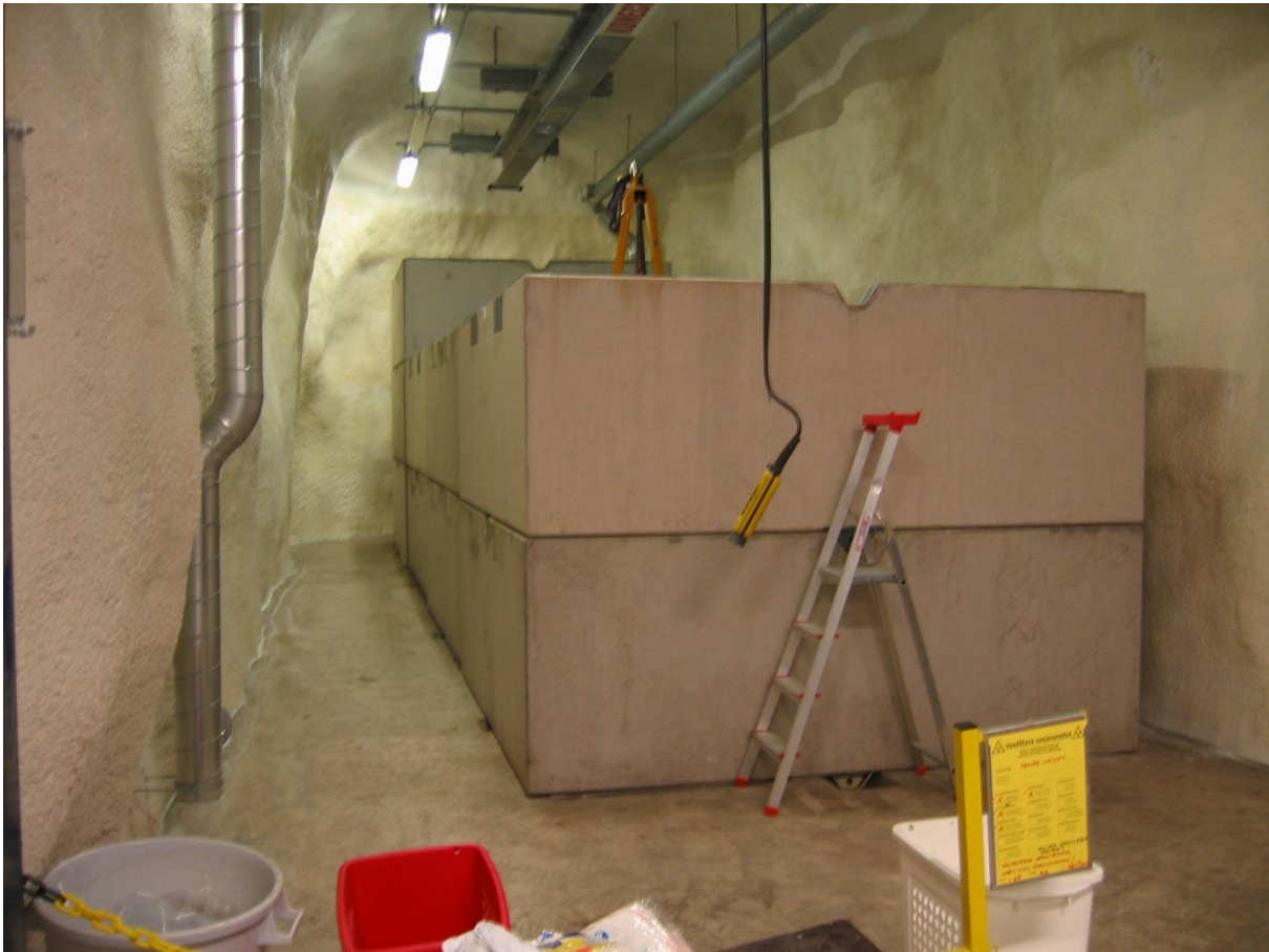
Figure 1 : Concrete containers, containing 16 bitumen waste drums, disposed in a concrete lined vault. Courtesy of TVO.
