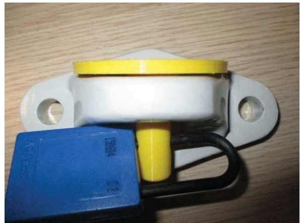
Figure 2: Tagged-out Tie-Off Point
